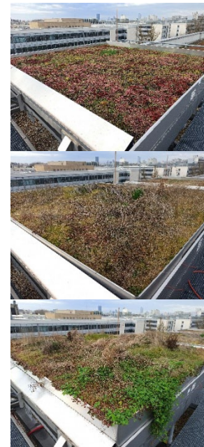
Figure 3. State of vegetation in Feb. 2025. Top to bottom: STR, MOS and GED.
